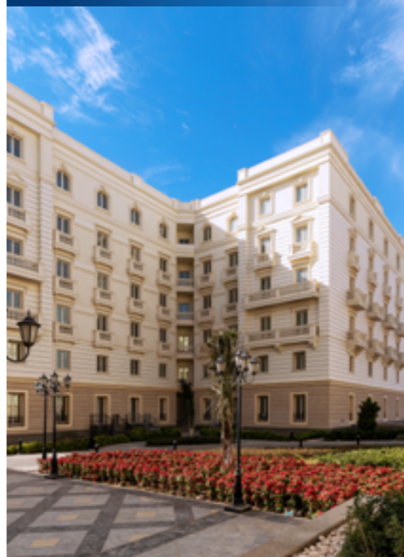
R5 Apartment Buildings
